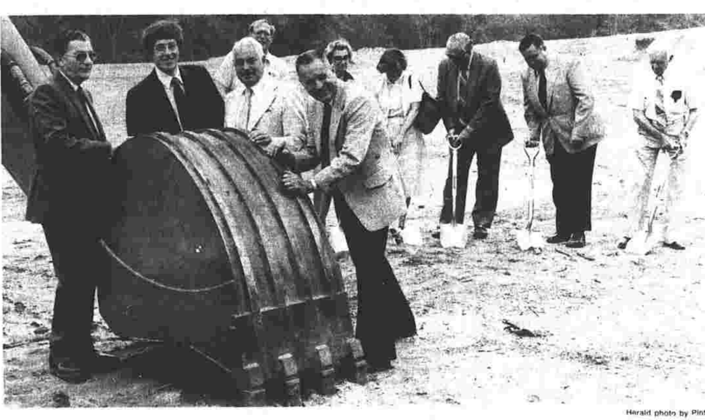
Moving dirt for cleaner water
